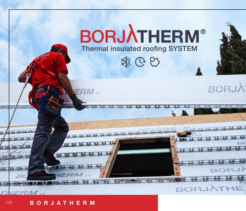
**BORJATHERM** panels are light-weight and easy handling, although to very easy to install. These panels make unnecessary most of the products which used to be essential for the construction of a ventilated roof because the panel itself, installed directly onto the rafters, beams or inclined slabs, performs all the functions of these products in one.
