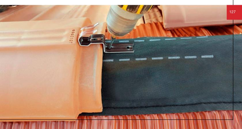
There may be joints between the roof and upper or lateral walls or around chimneys and other roof pipes. Adequate sealing of these joints must be done using Multi-use Waterproofing Flashing Tapes because these are critical points to ensure the correct roof waterproofing.
