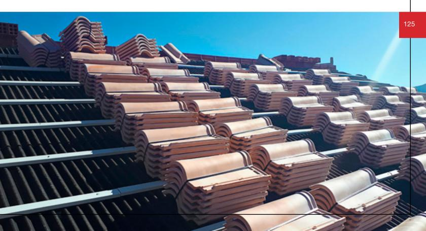
The first batten to be installed at the eaves must be at least 2 cm. higher than the rest of the battens to maintain the roof pitch in the first row of tiles. To achieve this additional height, a higher batten can be used, or an Eave comb + batten can be also installed on the first batten line.
