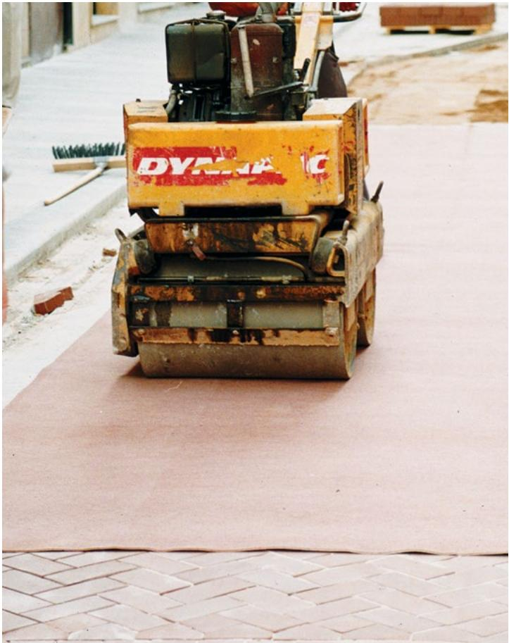
Compacting pavers. Use vibrators with rubber bases, or spread out a blanket as shown in the photo to avoid chipping.
