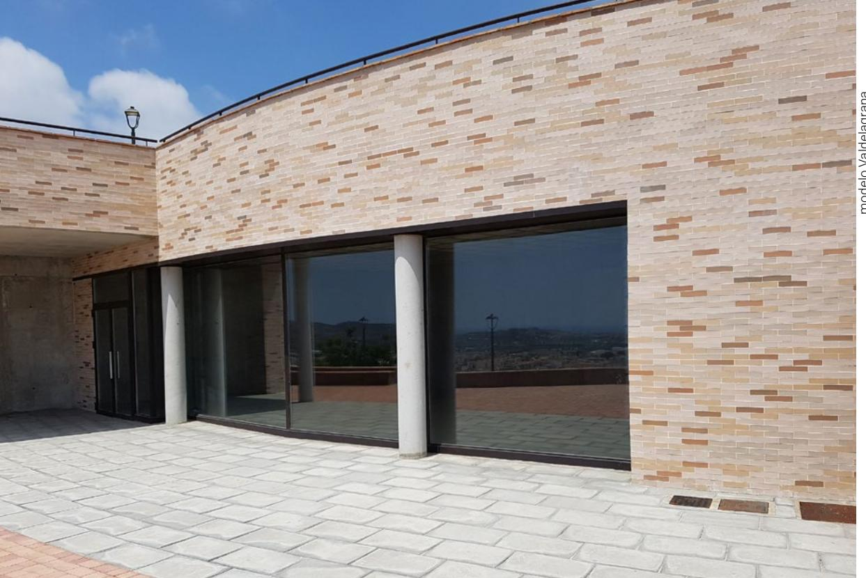
Ladrillo Extrusionado • *Extruded Brick*
