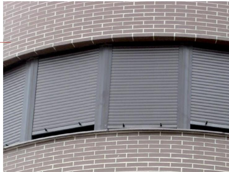
*In the brick factory wall hollows, the loader can be replaced by reinforcements in the courses located in the hollow lintel. The ceramic pieces are made with dovetail-shaped profiles, so that the good fixing of the pieces is favored. These pieces are designed to be placed on ropes, so as to provide continuity effect in the course immediately above the gap.*
