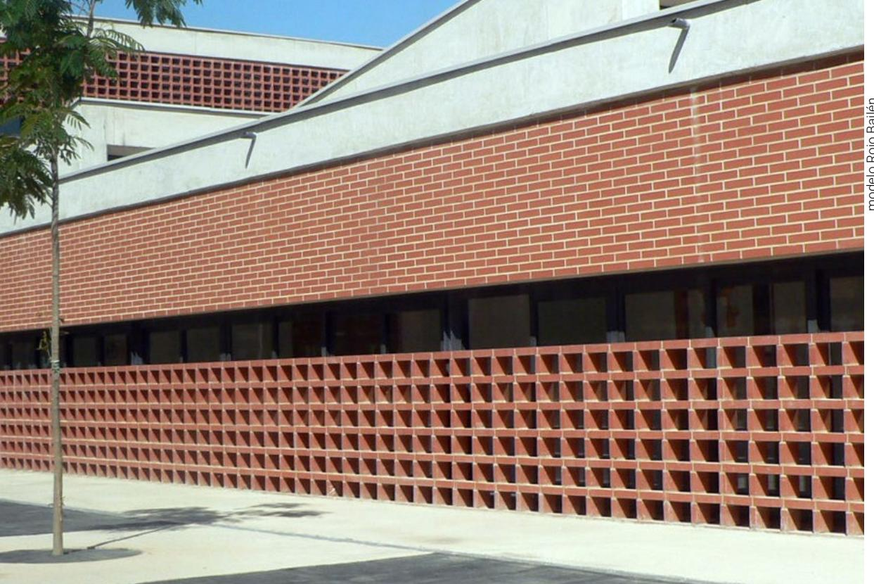
Ladrillo Extrusionado • *Extruded Brick*
